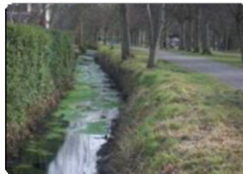
A canalised drainage ditch.
