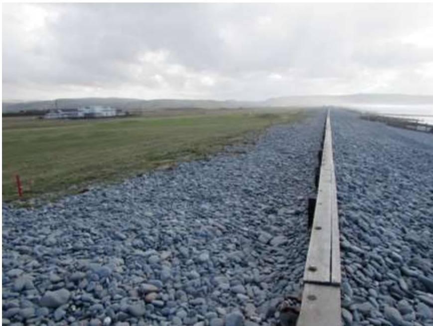
Figure 52 Timber revetment and groynes, Borth and Ynyslas Golf Club frontage, Ceredigion
