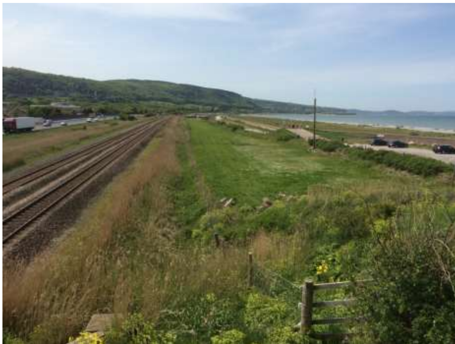
Figure 39 High value assets inland of the shingle beach at Pensarn, North Wales coast: from left to right are the A55 trunk road, the Chester to Holyhead railway line and a caravan park access road
