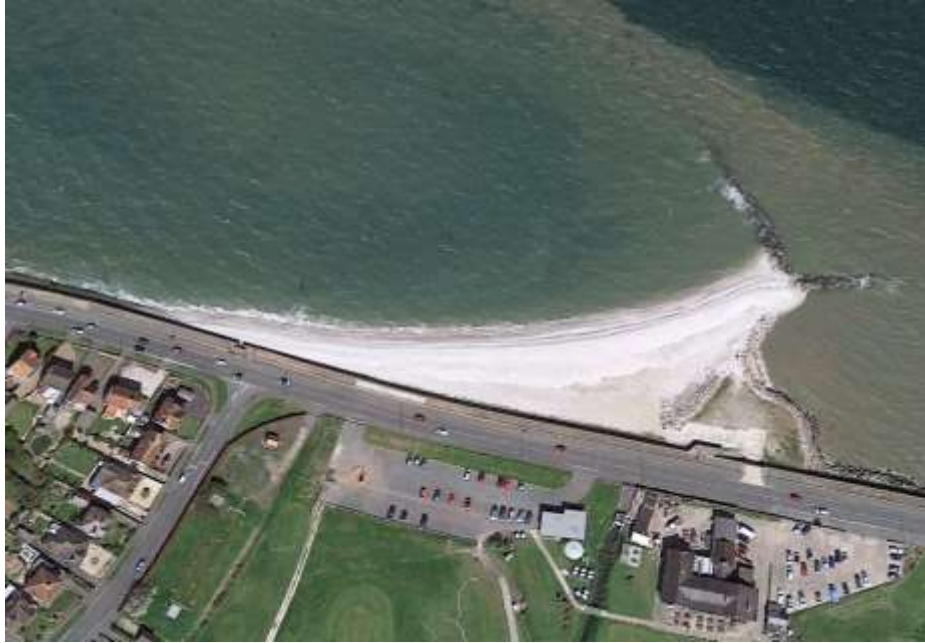
Figure 49 A fish-tail rock groyne and replenished beach at Penrhyn, North Wales
