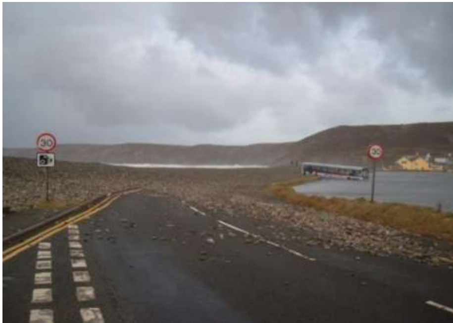
Figure 68 Storm overwash of the coast road at Newgale during the 2013-14 winter (photograph by Pembrokeshire County Council)
