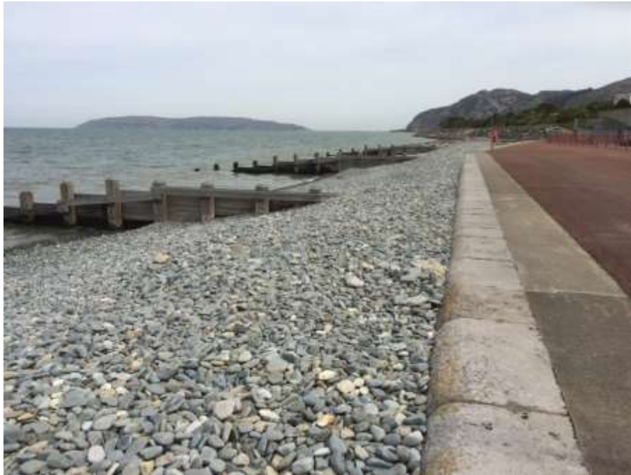
Figure 47 An example of effective timber groynes in front of Lanfairfechan promenade
