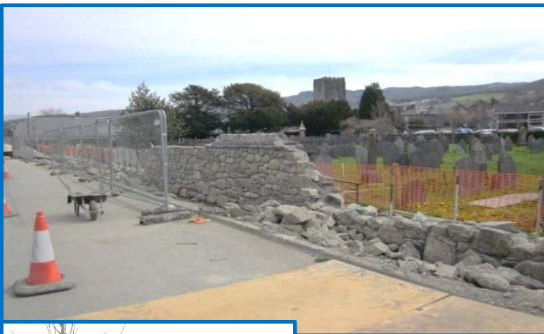
Fig 9 – construction of new flood defence wall set back from the river
