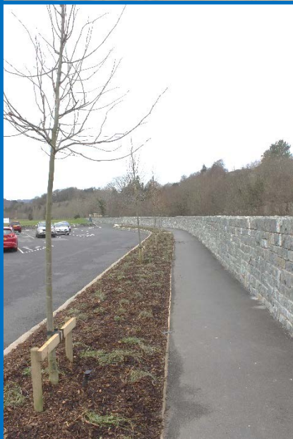
Fig 10 – Completed new flood defence wall along the Marian Mawr carpark
