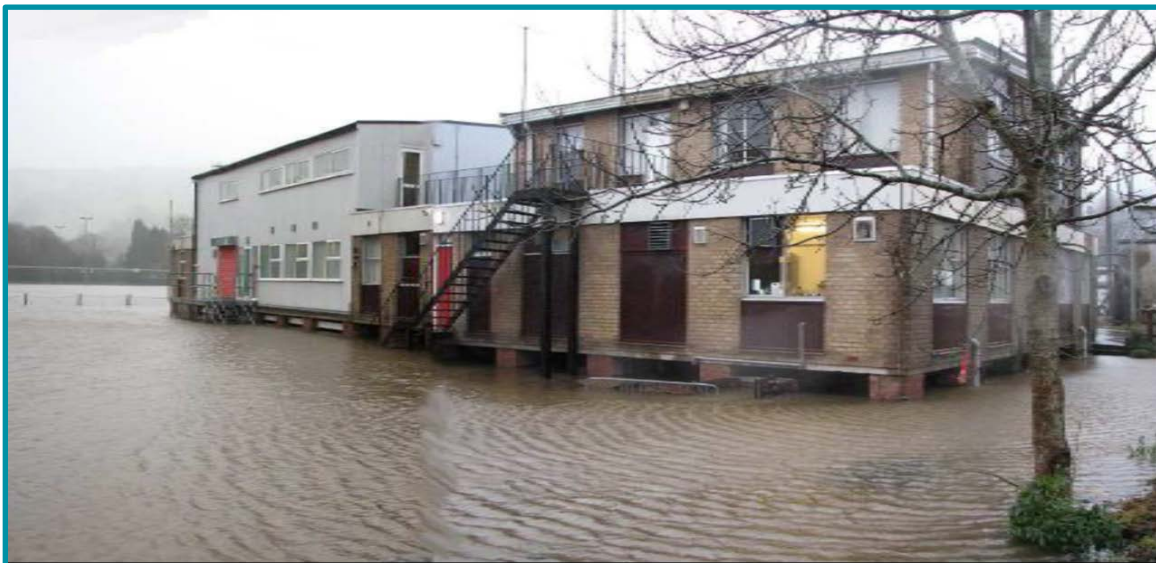
Fig. 10 below , Flooding to the rear of Dolgellau Fire Station, November 2009.
