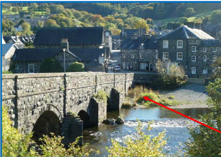
Fig 9 – View of deposition occurring at Bont Fawr bridge
