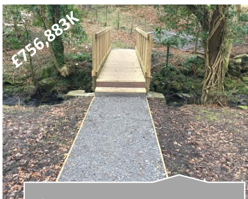
a) Practical improvements on the ground
