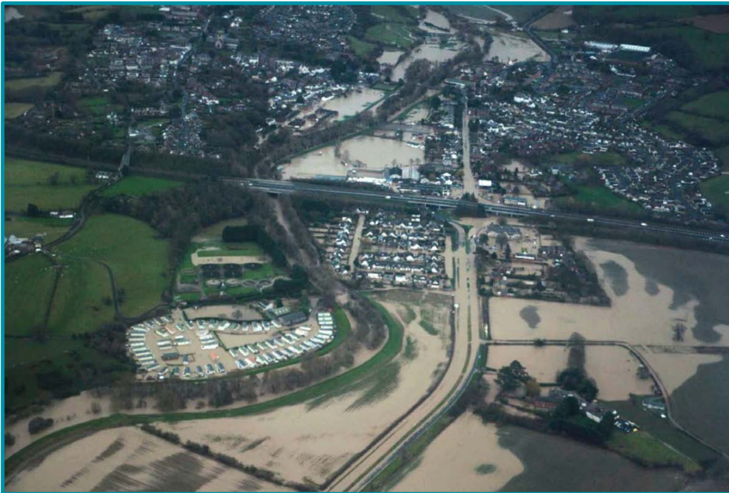
Figure 5 – photo demonstrating the breadth of flooding at St.Asaph
