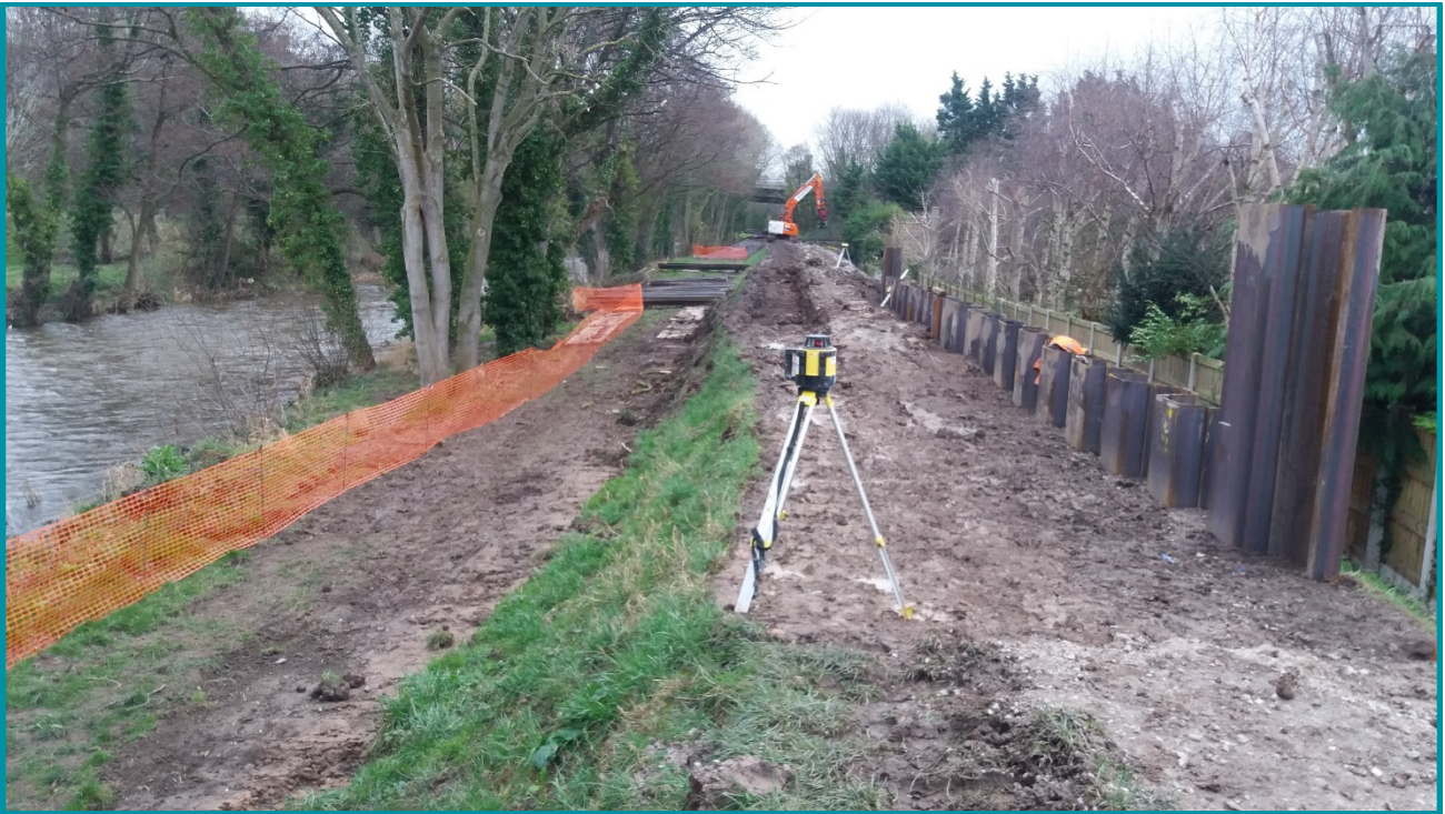
Figure 11 - several trees had to be removed along the river corridor to allow access for machinery to begin work on raising existing defences
