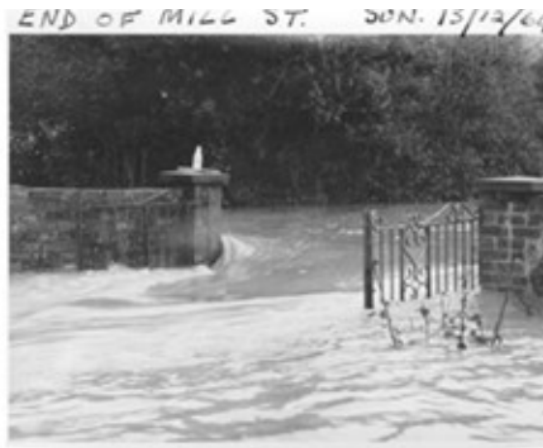
Figure 3 - Images from the 1964/1965 St.Asaph floods
